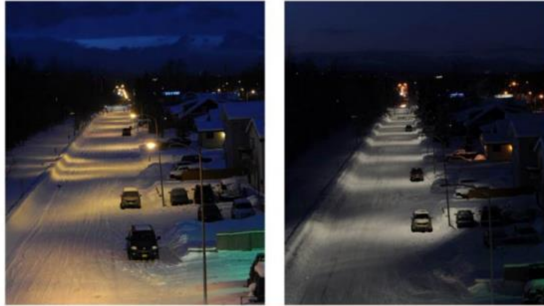
Figure 19. Photos. Images showing surround ratios from LED lighting (right) and traditional lighting sources (left) (Image Credit: DMD).
